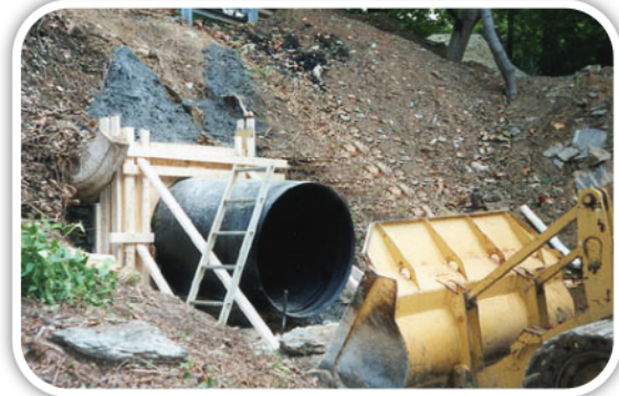
Cast in place headwall
