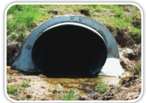
A culvert, rehabilitated with Snap-Tite® oval pipe.
