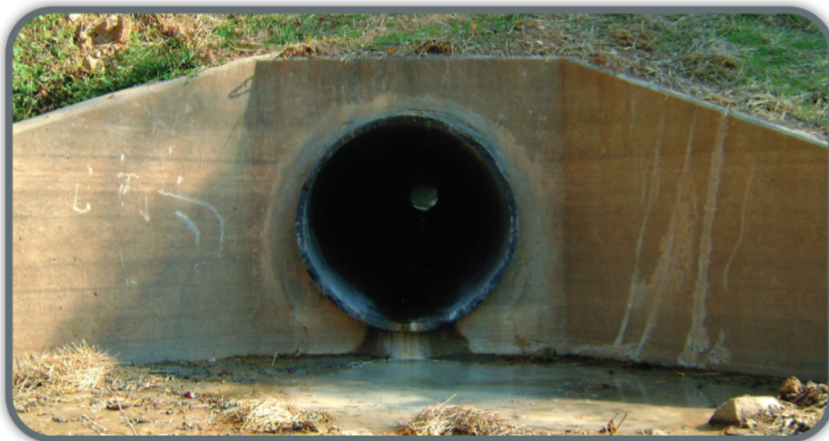
After rehabilitation with Snap-Tite®
